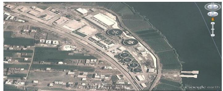
Figure 1 Aerial Diagram of Zifta Drinking Water Treatment Plant (ZWTP)
