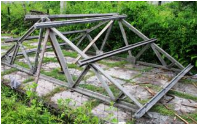
Fig.7. Finished roof truss system
