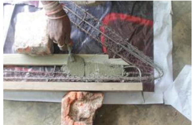
Fig.5. Laying of cement mortar
