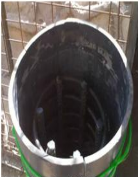
Figure ( 3 ) : Steel Reinforcement Cage in Plastic Tube Form
