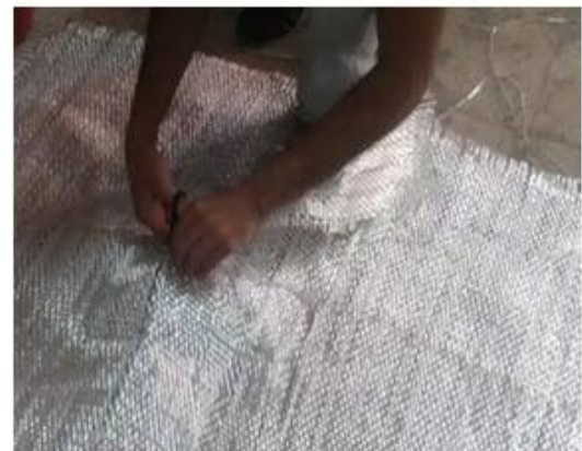
Figure ( 6 ) : Cutting The GFRP Wraps to Required Strips and Jackets
